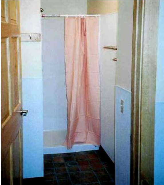
Camp Jewell YMCA, CT – FRP wainscot, mildew-free pastel paint for warmth, one-piece shower, 6-panel door (with a separate one for the toilet), sinks are in the hallway, tile floor, hooks and shelves and a resin stack-chair.
